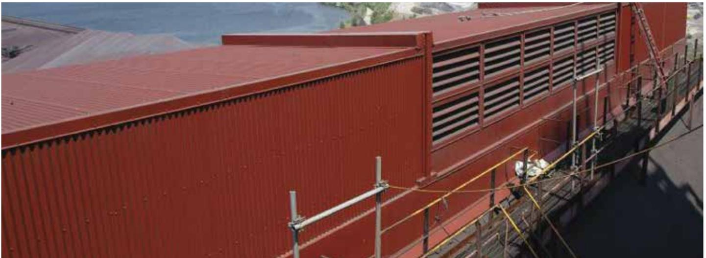
Completed at the end of June this year, the cladding was roll-formed and supplied by Agway Metals Inc. and installed by Lancaster Sheet Metal Ltd.
