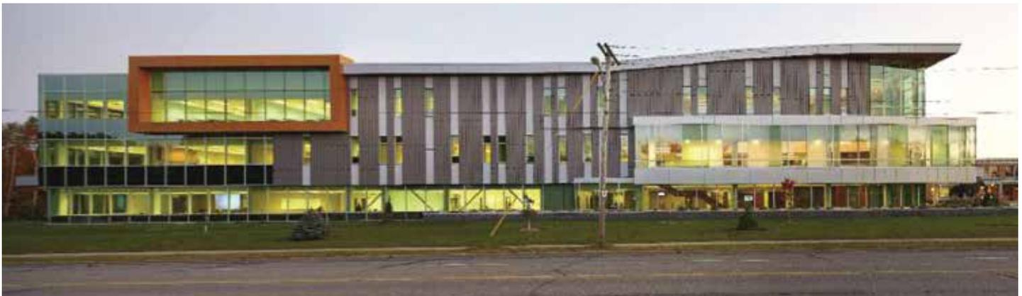
As can be seen in this photograph of the Academic Building, the predominate vertical steel cladding panels are Agway Metal's HF-IINF panels, coloured Grey Berry QC3659, while the narrower vertical panels are Agway Metal's HF-15NF, coloured Pebble QC3661, all with the 10000 Series paint system. (Agway's 7-175 panel is used on the penthouse, which is not visible in this view).
