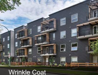
Wrinkle Coat is an organic, coated steel with a standard paint thickness of 35 or 40 microns. Architecturally attractive aesthetics with a mat finish that provides a unique wrinkled surface finish. The colours present a natural look and feel to the overall project.
