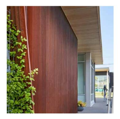
Gordon Maclean – the now-retired construction manager for the project – was in charge of artificially weathering the Indaten<sup>™</sup> steel before it made its way to the construction site. This was especially important for the portions of Indaten<sup>™</sup> that were used on the interior of the house.
