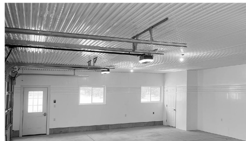
Residential applications like drivesheds, garages, and workshops
